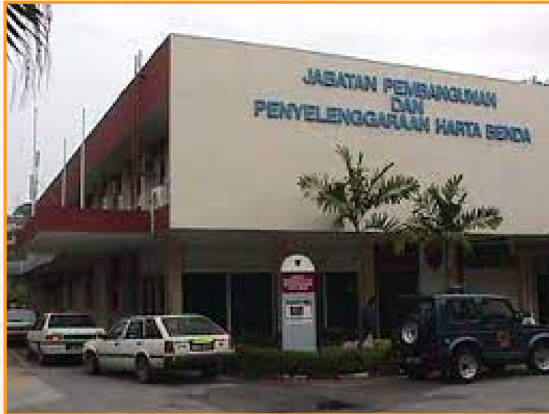
Photo: Department of Development and Estate Maintenance building
